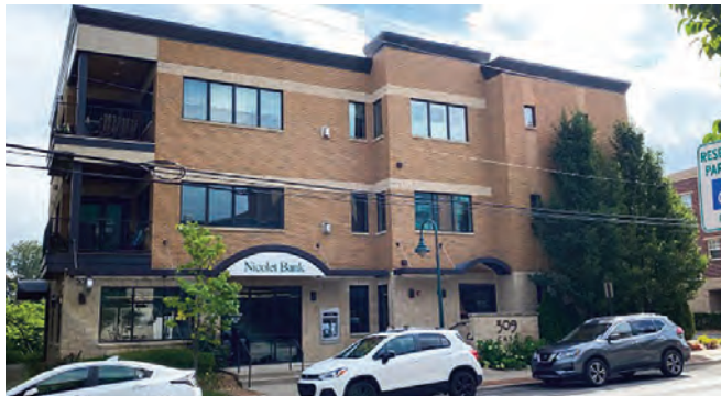
TRAVERSE CITY 309 Cass Street
